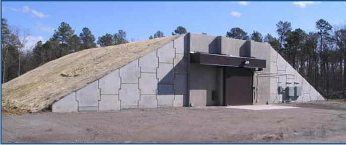
Construction of the first of five munitions supply buildings to securely store small arms, Fort Lee VA
